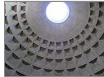
The oldest known concrete shell, the Pantheon in Rome , was completed about AD 125, and is still standing
