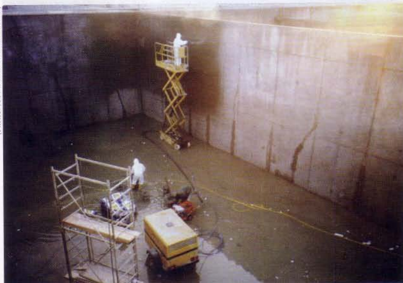
Figure 2 below right: Spray application works in the concrete basins.
