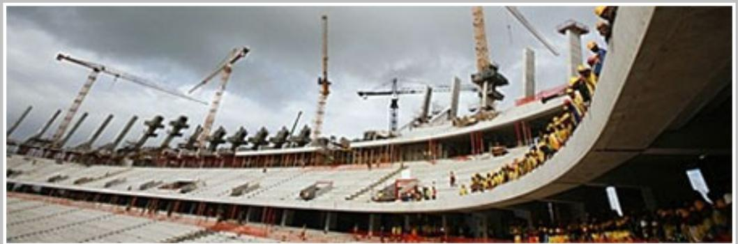
In order to effectively protect and waterproof the concrete in the seating stands, Penetron Admix was selected to treat the stitching between the precast seating. Therefore a total of 1100m<sup>3</sup> of concrete treated with Penetron Admix was poured on this iconic project site.
