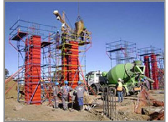
Penetron Admix was specified in 28 000 cubic metres of concrete in the public areas to strengthen the concrete and prolong the life of the building. It is thus a waterproof and maintenance-free facility.
